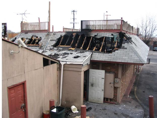
The two additions had wood frame roofs which abutted the original building's façade. The roofs were covered with standard asphalt shingles. See Figure 1 for the floor plan.
