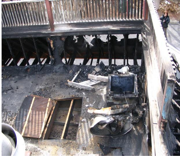
The fire spread from the ventilator to the back side of the building's decorative façade. The fire burned into the void space within the façade, and spread around the entire façade.
